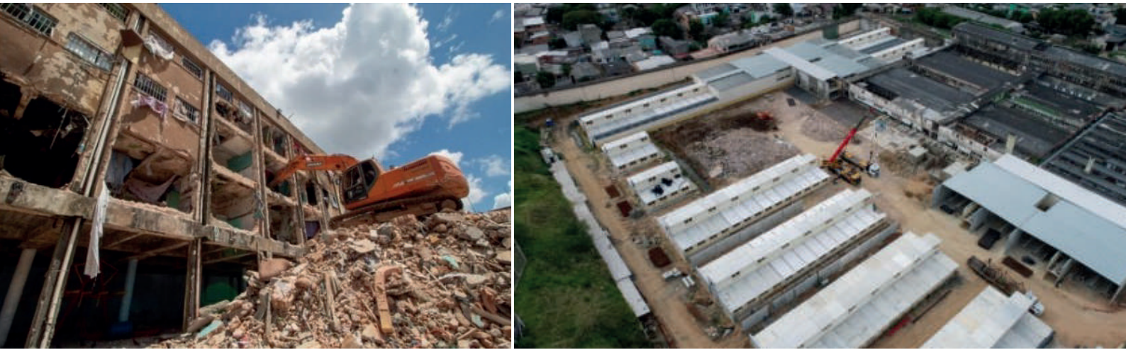
Figure 47 - Demolition of the old pavilions and assembly of the new modules at the CPPA
