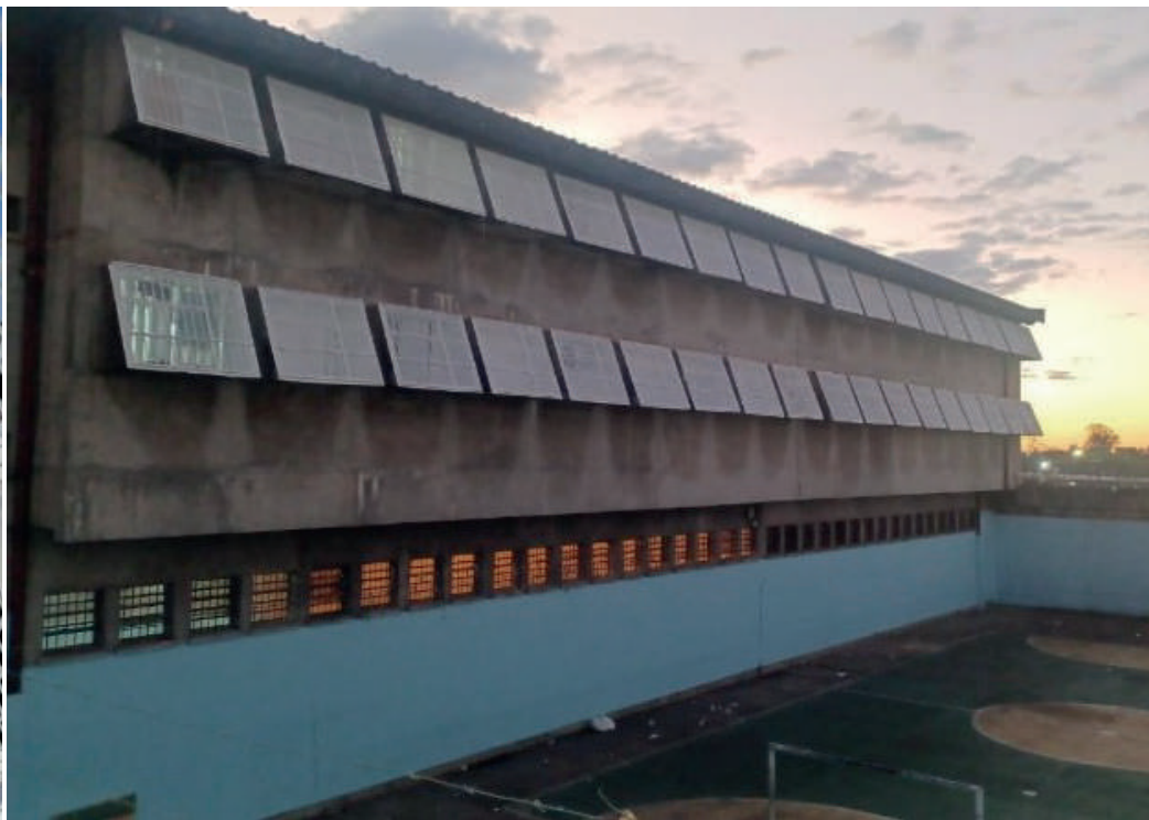
PASC with the pavilion windows screened
